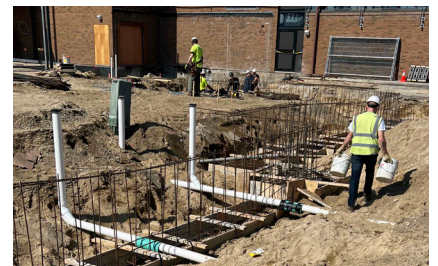
Above: Remainder of perimeter foundations at Area B.
