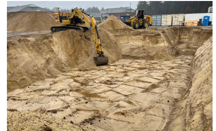
Above: Excavation for subsurface water chamber system.
