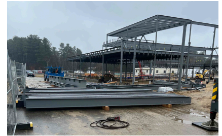
Above: Steel erection at Area B (Gym and Kitchen area).
