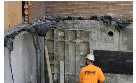
Above: Removal of old pump system under previous gym storage space.
